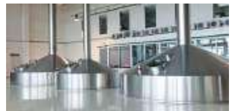
Brewery production equipment
