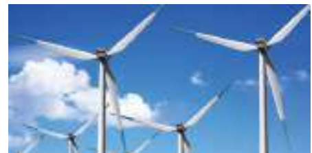
Wind turbine speed monitoring
